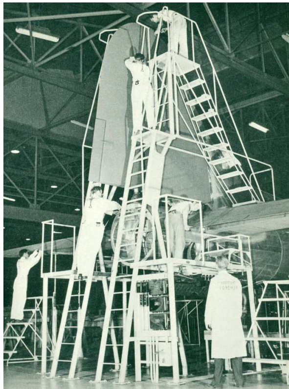
The vertical fin and horizontal tail being attached to a B-17E in the Boeing plant, early 1942.
