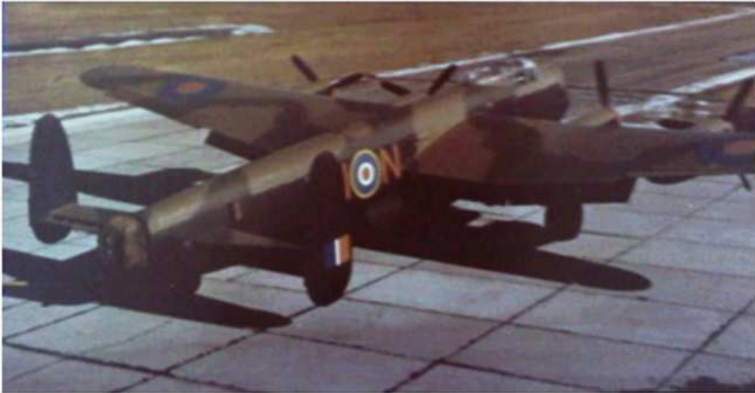
Garrison image after the completed paint job
